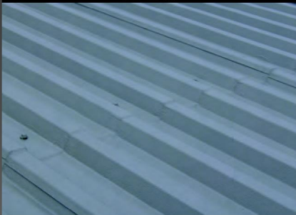
Plastisol® roof AFTER
